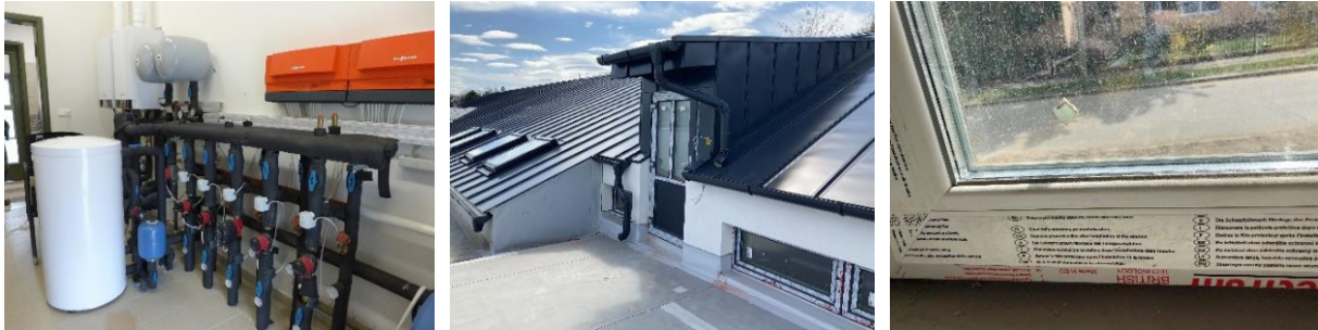
19. Figure - NESICA project building survey images
