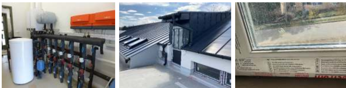
19. Figure - NESICA project building survey images
