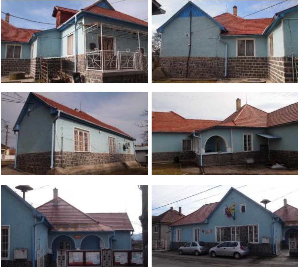
Figure 13 Views of building
