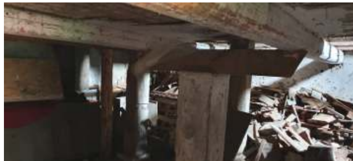
The House of Culture-City Library of the Liteni town. Roof structure
