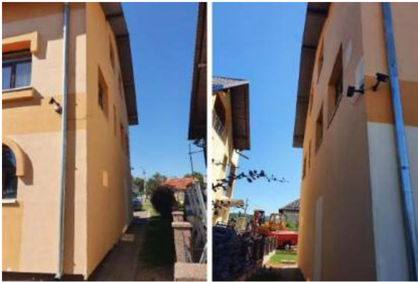
The rear facade of the City Hall building, Șcheia
